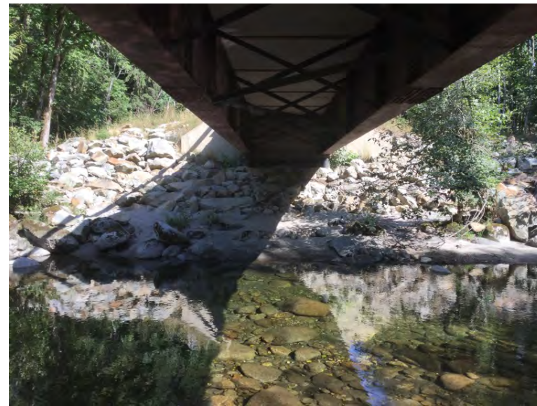
Right Bank Abutment when facing downstream
