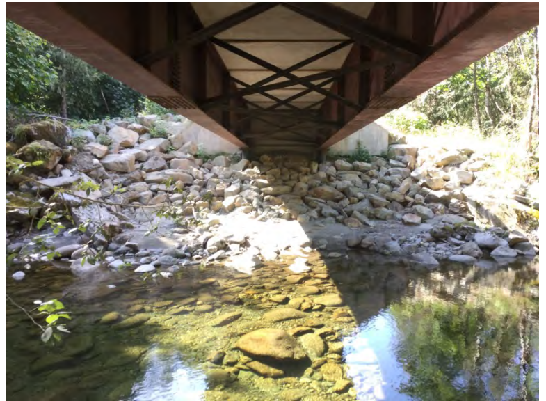
Left Bank Abutment when facing downstream
